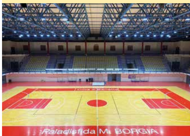
TRAVATURA METALLICA METAL STRUCTURE
